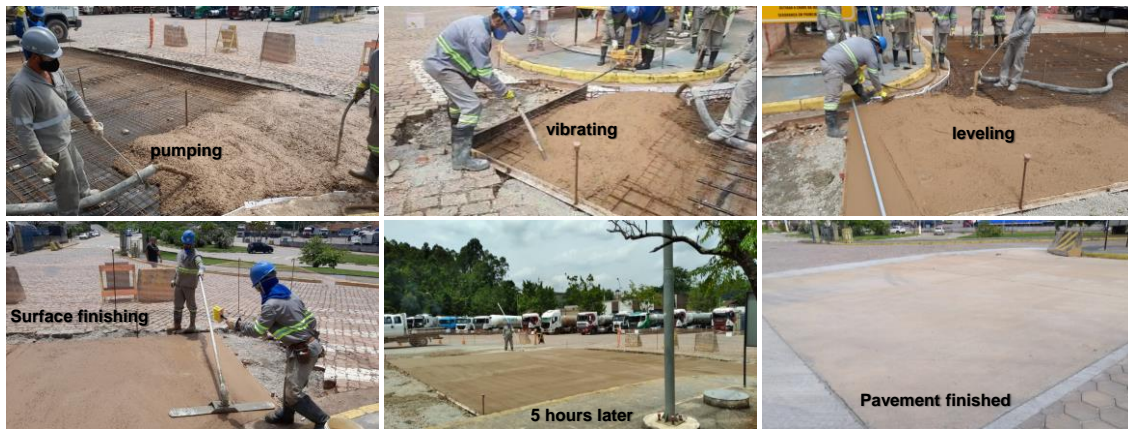
Figure 4. Stages during the production of the pavement using monolithic concrete.
