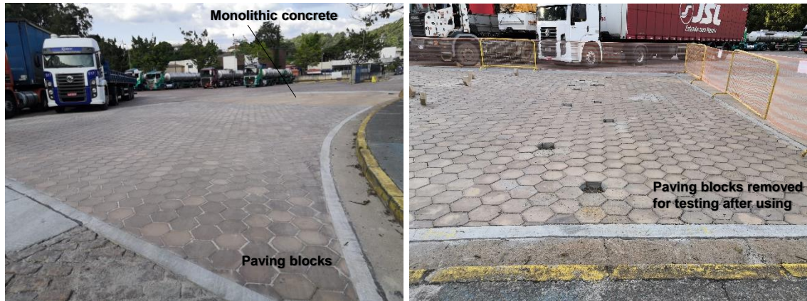
Figure 7. Pavement with paving blocks and with monolithic concrete.
